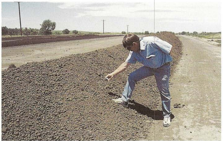
Plant Superintendent Kevin Clark taking windrow temperatures.
